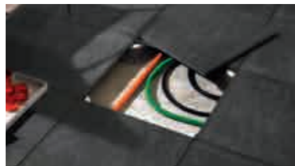
2. POSA SOPRAELEVATA. LAYING AS RAISED PAVING.
