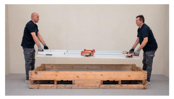
**3.** Lift the slab gently and place it on the workbench, or turn it to the vertical position and place it on the handling trolley for adhesive application.
