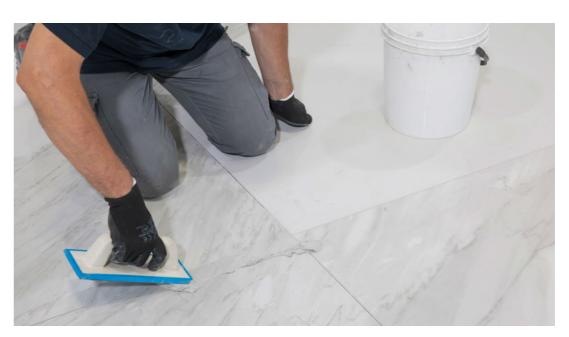
**8.** Alternate and lay out the pieces to create a natural distribution of the pattern and grains. We suggest to match grout colour with slab, using a minimum space of 2 mm when laying a single size (as foreseen by European regulation).
