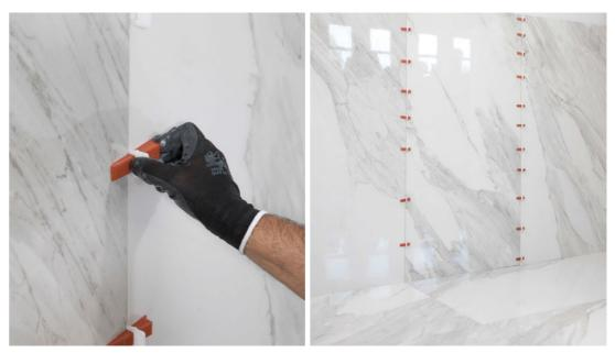
7. As with all large-sized tiles, levellers should be used to ensure the very best result in terms of appearance.
