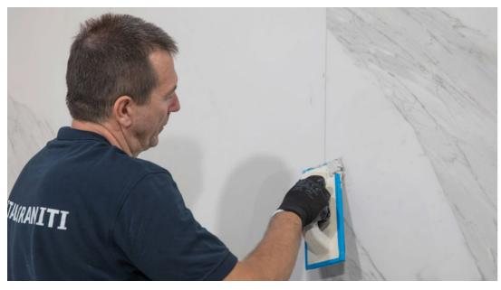
**8.** Alternate and lay out the pieces to create a natural distribution of the pattern and grains. We suggest to match grout colour with slab, using a minimum space of 2 mm when laying a single size (as foreseen by European regulation).
