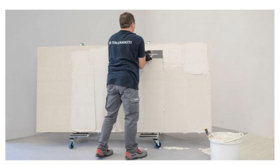
**4.** Apply the adhesive to the back of the slab using the serrated trowel with square teeth (3x3 mm) and make sure that the adhesive lines in the slab run in the same direction as those created by the last pass of the trowel in the adhesive on the wall. During application, the slab should be vertical, secured to the handling bars / frame with safety suction cups placed on the wheeled transporter trolley.
