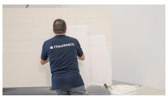
**3.** After applying the adhesive, make sure that all the lines created by the last pass of the trowel run in the same direction (theoretically, the lines should be parallel to the short side of the slab), taking care to avoid criss-cross lines, which tend to trap air in the centre of the slab.
