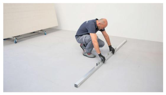
1. Before proceeding with final installation, check that the substrate is perfectly flat, dry and clean. Use the adhesives described, mixed in accordance with the instructions provided in the relevant technical information. High performance cement adhesives in class C2 or above should be used.
