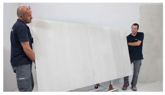
5. Use the handling bars / frame with safety suction cups to move the slab into position and lay it in place.
