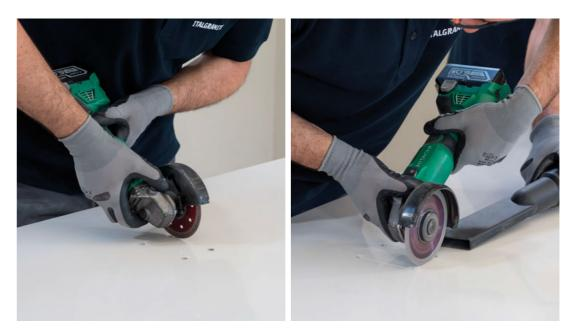
**3.** Cut the section between the hole and the end of the slab using an angle-grinder fitted with a diamond blade.
