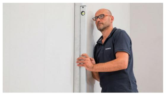
1. Before proceeding with final installation, check that the substrate is perfectly flat, dry and clean. Use the adhesives described, mixed in accordance with the instructions provided in the relevant technical information.
