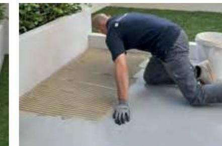
Clean the existing surface and check that the screed has been properly prepared: flat, dry and cured. Spread the adhesive evenly over the surface.
