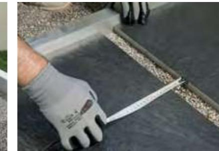
Place the slabs dry on the gravel and check that the gap between them is the same over the entire laying surface. Tap down gently with a rubber hammer to settle them into place and eliminate any unevenness.
