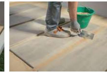
Add sand in the joints to level the paving. Clean the surface of the slabs.
