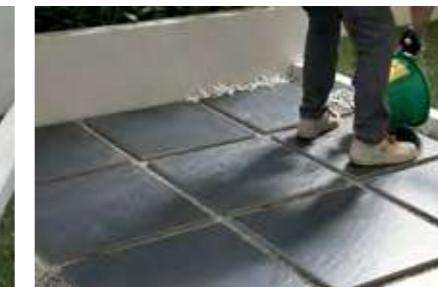
Check the flatness of the surface created. Add gravel in the joints to level the paving. Decorative gravel larger in diameter than the type used for the substrate can also be used in the joints.
