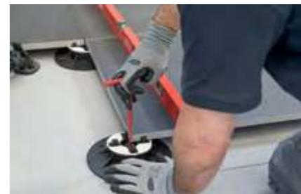
Lay the slabs on the pedestals dry. Add a pedestal in the middle of the slab, removing the spacer wings. Systematically check the flatness and adjust the heights of the pedestals with the adjuster key to compensate for any unevenness in the substrate. A little slope of the substrate is always recommended in order to prevent water stagnation underneath the surface.
