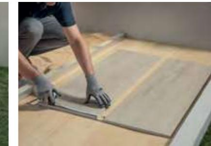
Place the slabs dry on the sand and check that the gap between them is the same over the entire laying surface. Tap down gently with a rubber hammer to settle them into place.
