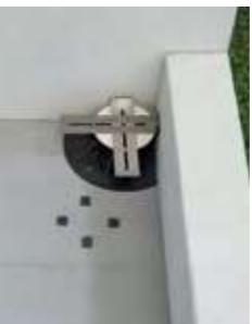
Arrange the grid of pedestals in accordance with the laying diagram, starting with those around the edge. Fit the protective tile edge clips on the pedestals against any walls.
