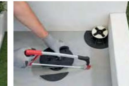
Clean the existing surface and check that the screed is level to select the right type of pedestal. The screed must be dry and cured. Prepare the chosen pedestals, cutting the ones around the edge to size and removing any unwanted wings.
