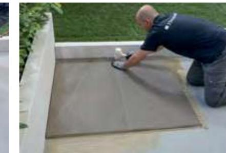
Put the slabs in place and tap down gently with a rubber hammer to drive out the air and ensure perfect bonding. Fit the 4/5 mm spacers into the joints.
