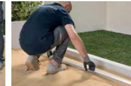
Prepare a layer of sand at least 5 cm thick on the existing substrate (screed or gravel). Level the surface with a straightedge and check the flatness.
