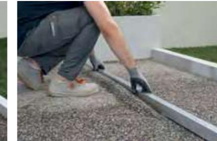
Create a layer of at least 5 cm of gravel (diam. 3/6 mm) on the existing substrate. Level the surface with a straightedge and check the flatness.
