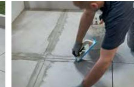
Once the glue has dried, remove the spacers, grout the joints and clean thoroughly to remove any residues.
