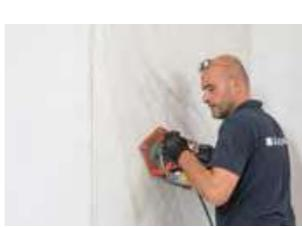
IT 6. Use a vibrator for tiles (or alternatively a cushioned plastic hammer) to make sure that the slab is glued evenly to the substrate. Tap from the centre to the edges to assist the venting of any air pockets between the slab, the adhesive and the substrate. Do not use hammers or unsuitable tools.
