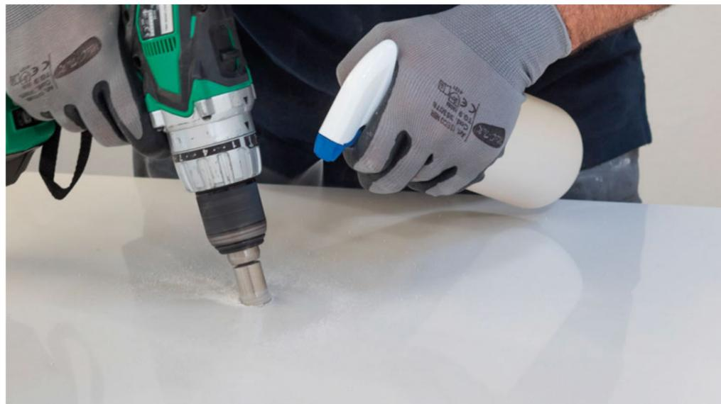
2. Drill the hole at an angle of 75°-85° to a depth of 1-2 mm into the slab.
