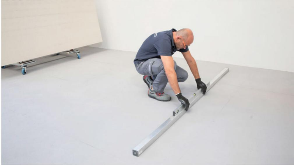
**1.** Before proceeding with final installation, check that the substrate is perfectly flat, dry and clean. Use the adhesives described, mixed in accordance with the instructions provided in the relevant technical information. High performance cement adhesives in class C2 or above should be used.
