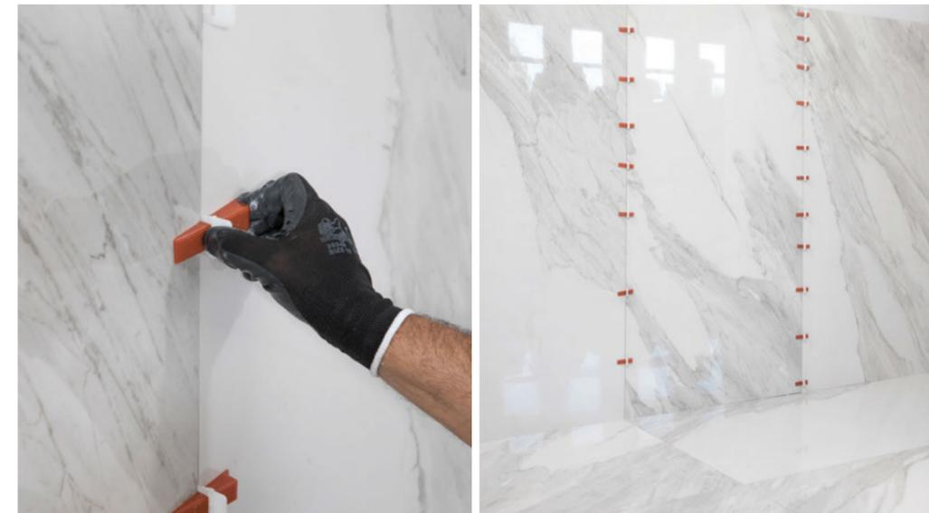
7. As with all large-sized tiles, levellers should be used to ensure the very best result in terms of appearance.
