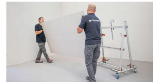
Handling trolleys designed to allow application of adhesive to the back of the slab.
