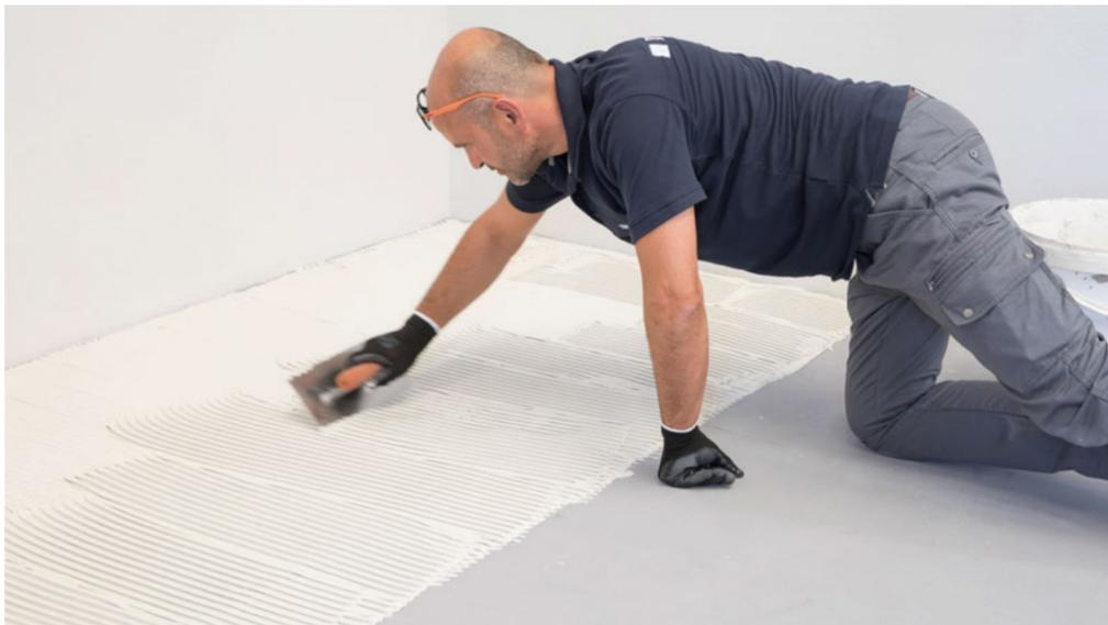
**2.** Apply the glue to the floor using a serrated trowel with slanted teeth (10x10 mm), spreading the adhesive 5/10 cm beyond the edges of the slab.
