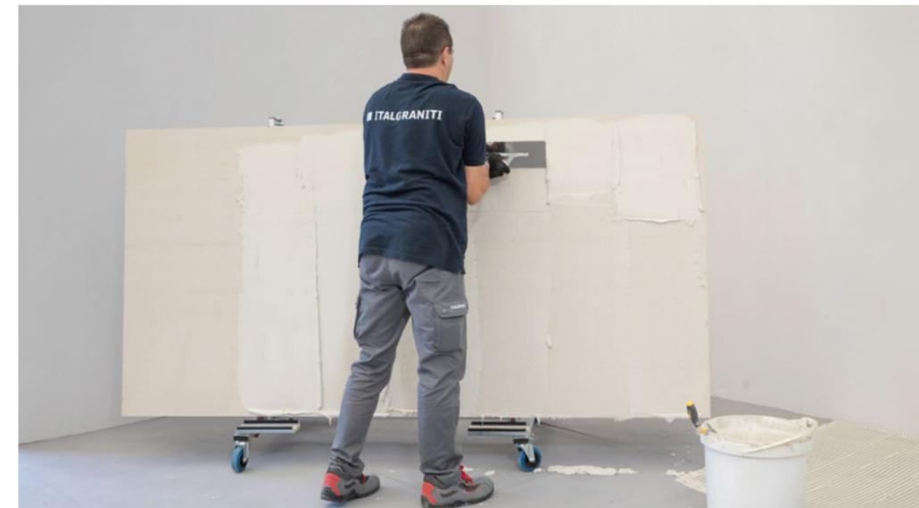
**4.** Apply the adhesive to the back of the slab using the serrated trowel with square teeth (3x3 mm) and make sure that the adhesive lines in the slab run in the same direction as those created by the last pass of the trowel in the adhesive on the wall. During application, the slab should be vertical, secured to the handling bars / frame with safety suction cups placed on the wheeled transporter trolley.
