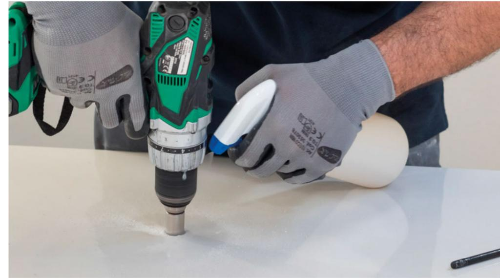
3. Keep the drill/screwdriver at an angle of 90° and, applying gentle, constant pressure, make circular movements at an angle of about 5°-10°. Do not push the drill/screwdriver straight downwards and make sure that there is sufficient water to keep the tool wet throughout the procedure.
