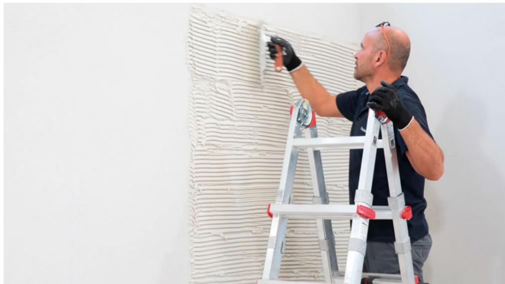
**2.** Apply the glue to the wall using a serrated trowel with slanted teeth (10x10 mm), spreading the adhesive 5/10 cm beyond the edges of the slab.
