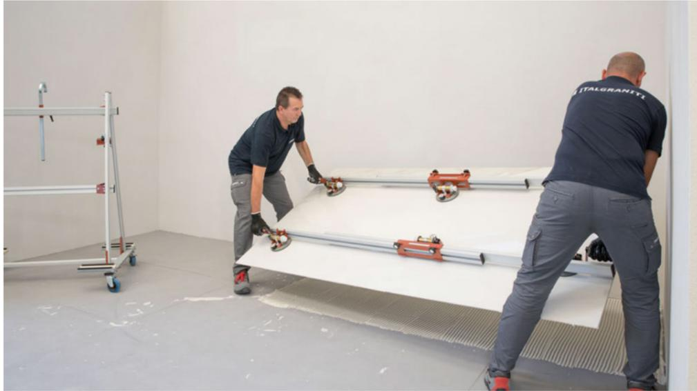
5. Use the handling bars / frame with safety suction cups to move the slab into position and lay it in place.
