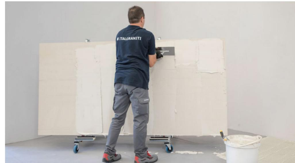
**4.** Apply the adhesive to the back of the slab using the serrated trowel with square teeth (3x3 mm) and make sure that the adhesive lines in the slab run in the same direction as those created by the last pass of the trowel in the adhesive on the floor. During application, the slab should be vertical, secured to the handling bars / frame with safety suction cups placed on the wheeled transporter trolley.
